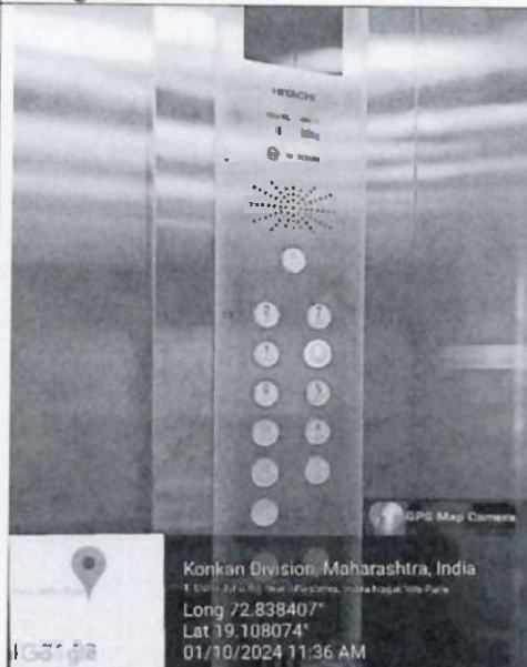
Elevator with Braille symbols, auditory signals, and emergency buttons
